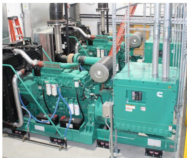
*Figure 2. Redundant generators ensure that storage temperatures are maintained in the event of grid power loss due to storms or other unplanned events.*
