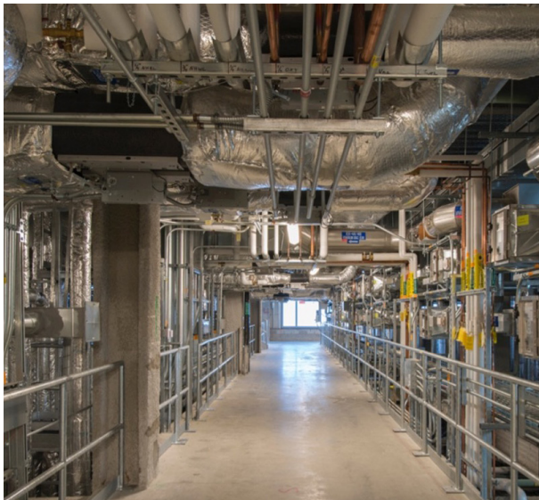
Interstitial space to house mechanical systems at UMass Medical School's Sherman Center.
