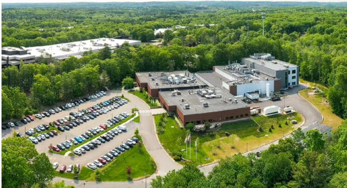
Manufacturing facility of Rentschler Biopharma in Milford, Massachusetts
