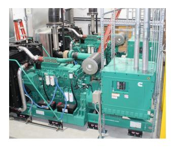
Figure 2. Redundant generators ensure that storage temperatures are maintained in the event of grid power loss due to storms or other unplanned events.
